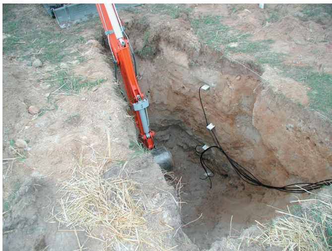
Figure 1. Installation of soil moisture probes at the Bemidji crude-oil spill site in Minnesota. Data from these probes are being used to estimate recharge based on the zero-flux plane method.
