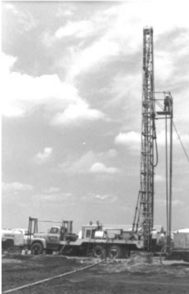
Drilling observation well.
