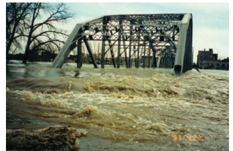
At the Sorlie Bridge between Grand Forks, N. Dak., and East Grand Forks, Minn., floodwaters from the Red River of the North crest at 54.35 feet, Tuesday, April 22, 1997. This depth was more than 24 feet above flood stage and more than 4 feet above the previous record. (USGS photo)
