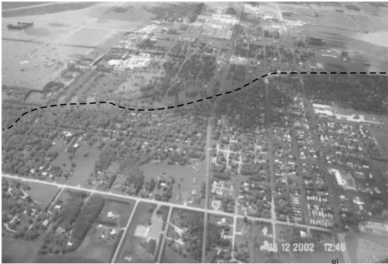
Roseau, Minnesota - June 12, 2002 - flooding from the Roseau River.
